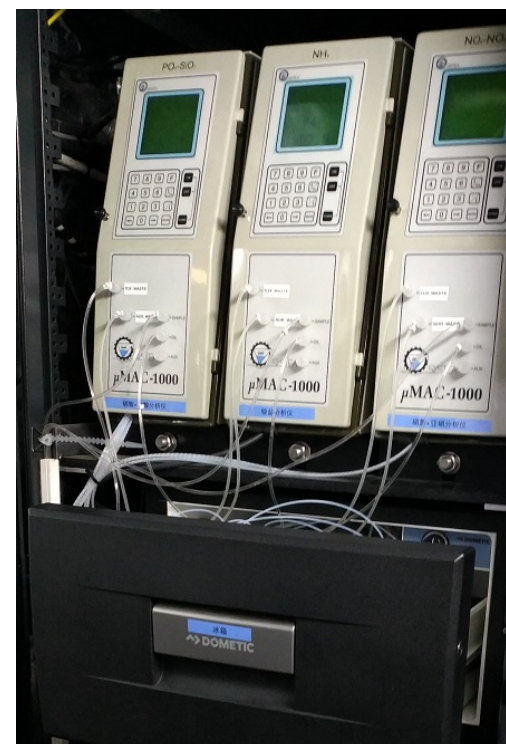
Ferry Box installation
