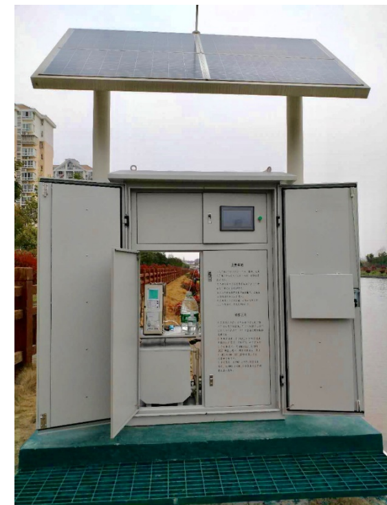
Self-powered Ministation for river water control
